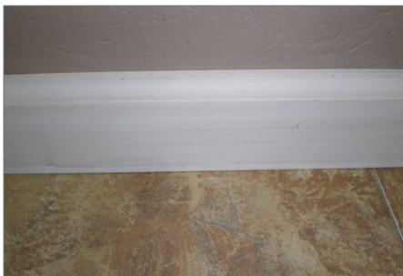
Ceramic with primed wallbase
