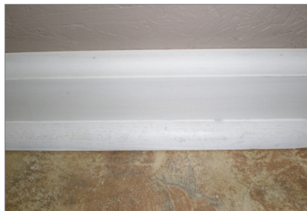
Ceramic with primed wallbase and quarterround
