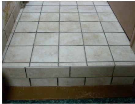
Step 2: Before grouting and sealing
