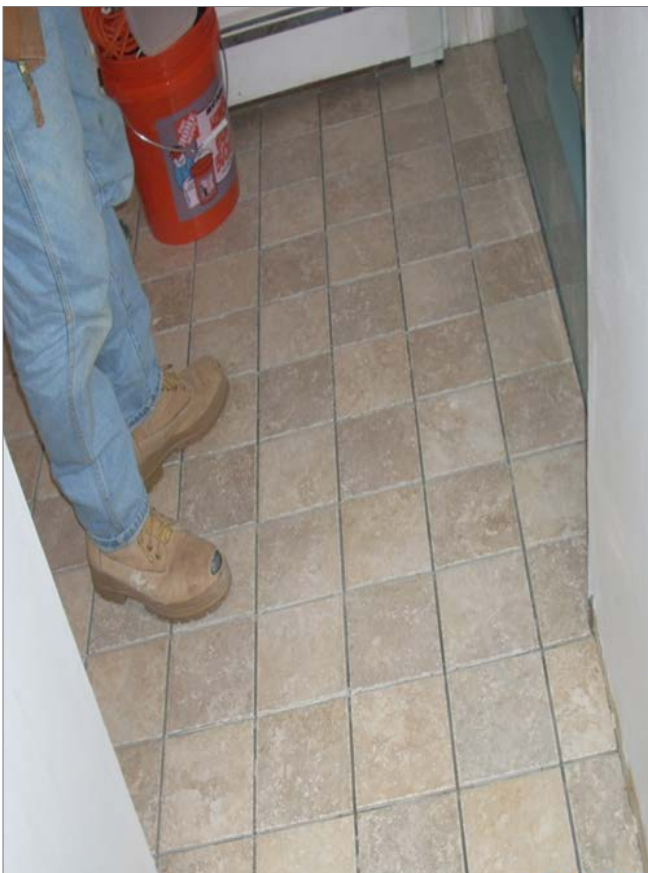
Before grouting, sealing and cleaning
