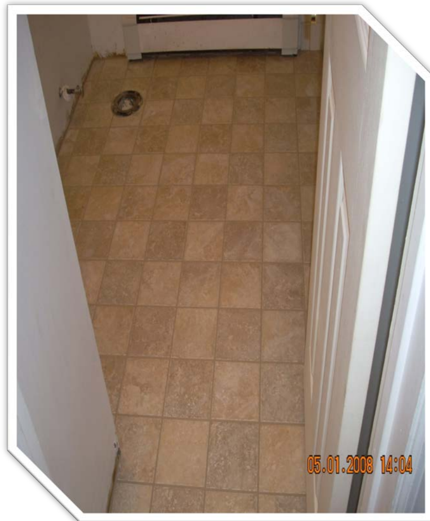
AFTER GROUTING, SEALING AND CLEANING
