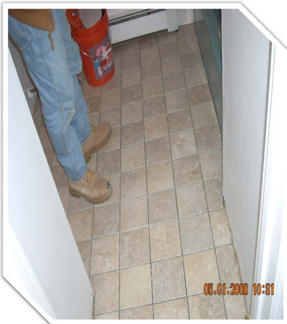
BEFORE GROUTING, SEALING AND CLEANING
