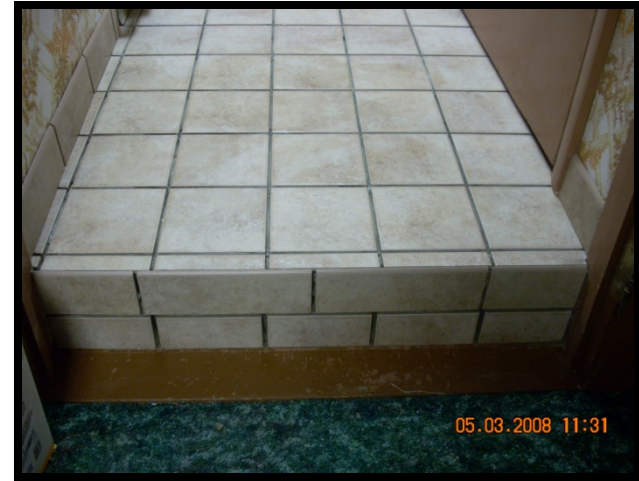
BEFORE GROUTING AND SEALING
